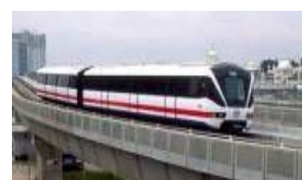
Kuala Lumpur LRT System 2 (Malaysia)
