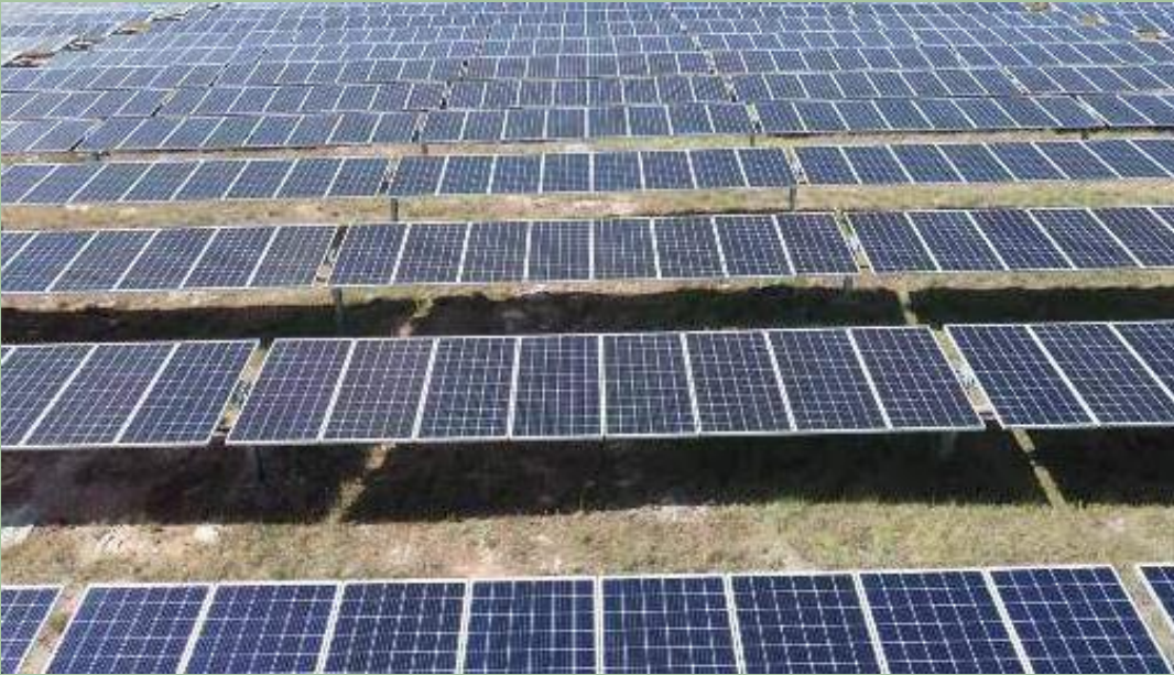
Stand-Alone Solar Home Systems
